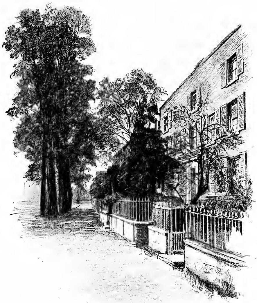
KELMSCOTT HOUSE, HAMMERSMITH, 1887
